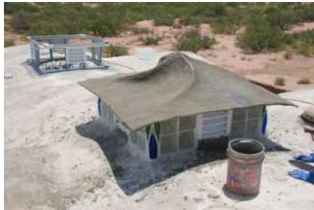
Dome Constructed out of Ferro-cement
