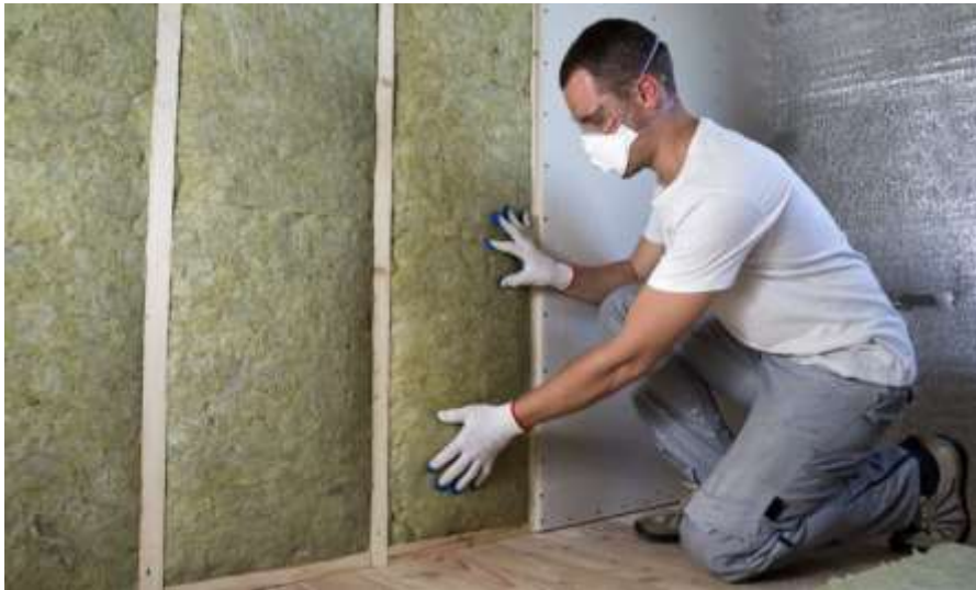
Images showing the use of thermocol sheets in walls
